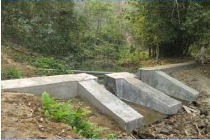
Water Harvesting structure at Amphreng
